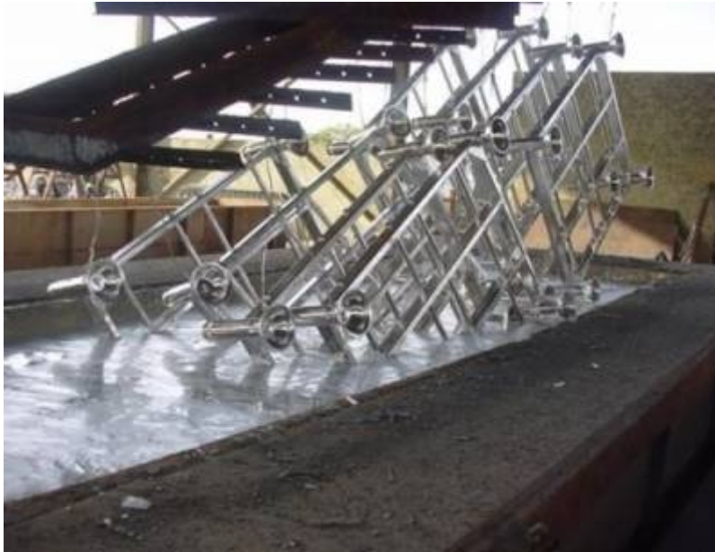
Figure 52: Hot dip galvanising
